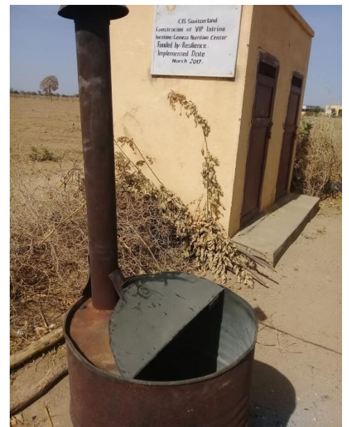
Rehabilitated latrine, Jemaiza
