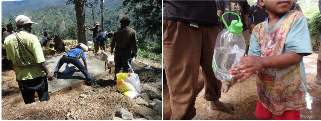
Photo on right: Tank base work in progress at Kangir
