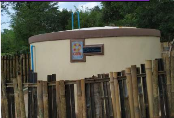
Water tank in Long Waun Village (Shan)
