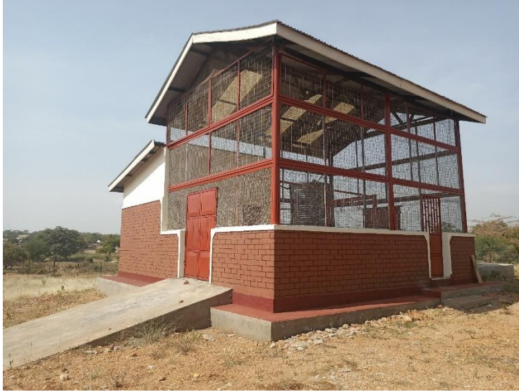
Renovated slaughter shade in Amudat district.
