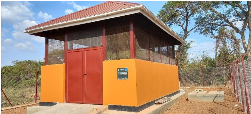
The completed slaughter shade in Toroma Town Council
