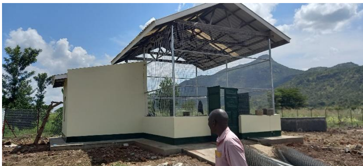
Completed renovated Town Council abattoir, Abim district.
