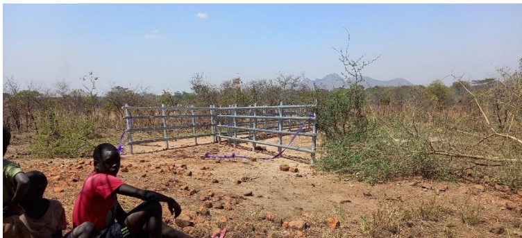
Completed cattle crush.
