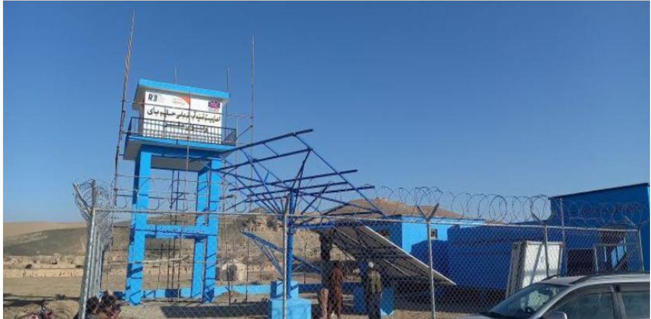
Figure 36 Kahm Abbasy Village, Muqur district. WVI and R3 logo displaced on new water installation
