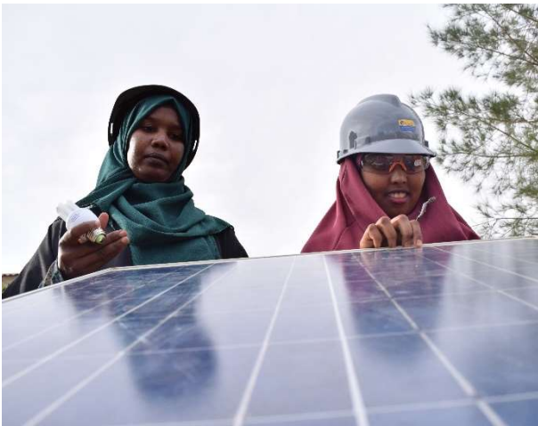
Installing solar panels in Somalia
