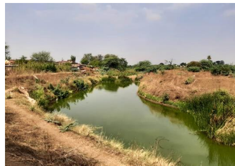
Picture 4 Water Harvesting Structure in Mendhla Village, Yavatmal (May 2021)
