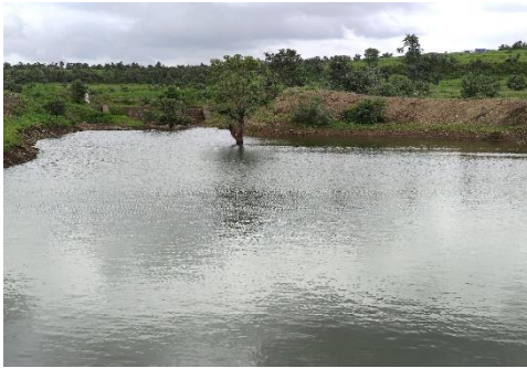
Picture 3 Water Harvesting Structure in Donoda Village, Yavatmal (August 2021)
