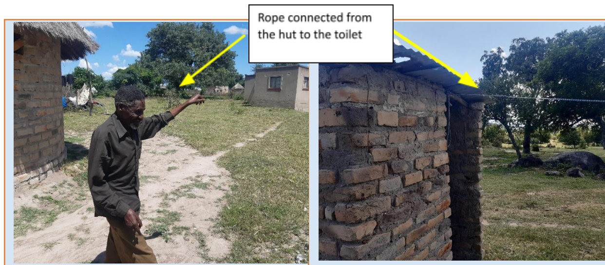
Plate 2: Innovative latrine with connecting rope for people with visual impairment and elderly persons
