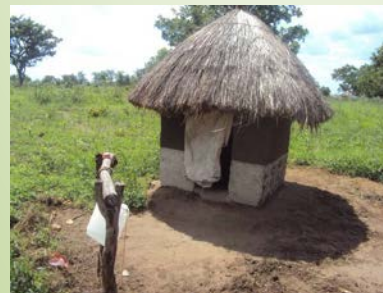
A constructed household latrine with hand washing facility (tippy tap) in Tetugu village
